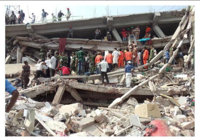
Rana Plaza after the collapsed. Photo taken from south side of building - Odhikar
